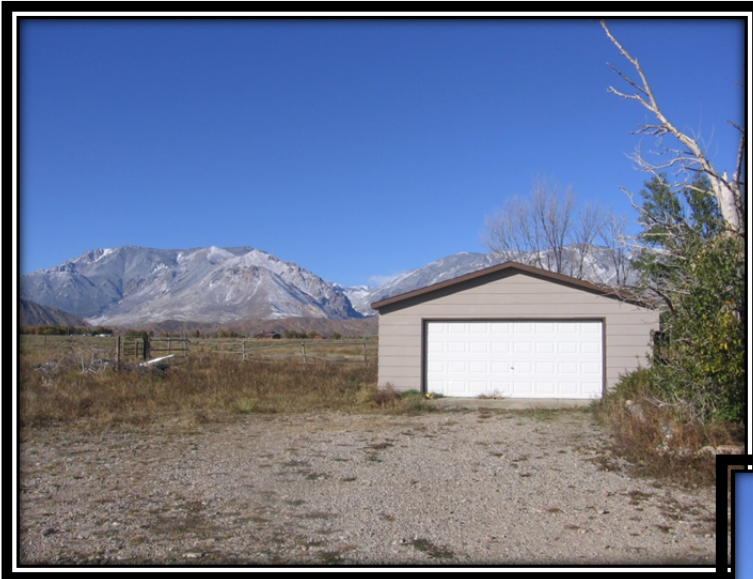
Garage & Mountain Views
